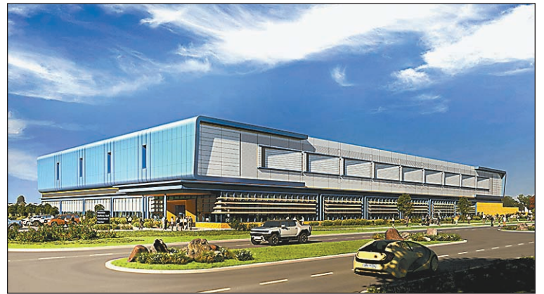
The Wallace Center, under construction at the GM Tech Center in Warren, is expected to accelerate new technologies like lithium-metal, silicon and solid-state batteries along with production methods that can quickly be deployed at battery cell manufacturing plants like GM's joint ventures with LG Energy Solution in Lordstown, Ohio, and Spring Hill, Tenn. photo: by GM
