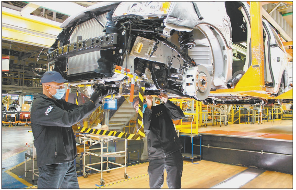
A weld curtain hangs between two operators working on the underbody of a Dodge Grand Caravan at FCA's Windsor (Ontario) Assembly Plant. The barrier helps protect employees from the spread and transmission of COVID-19.
