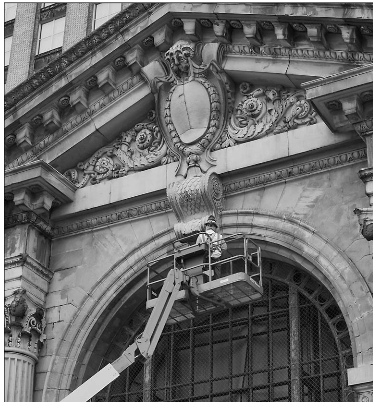
Ford has started the construction phase of its Corktown project.
