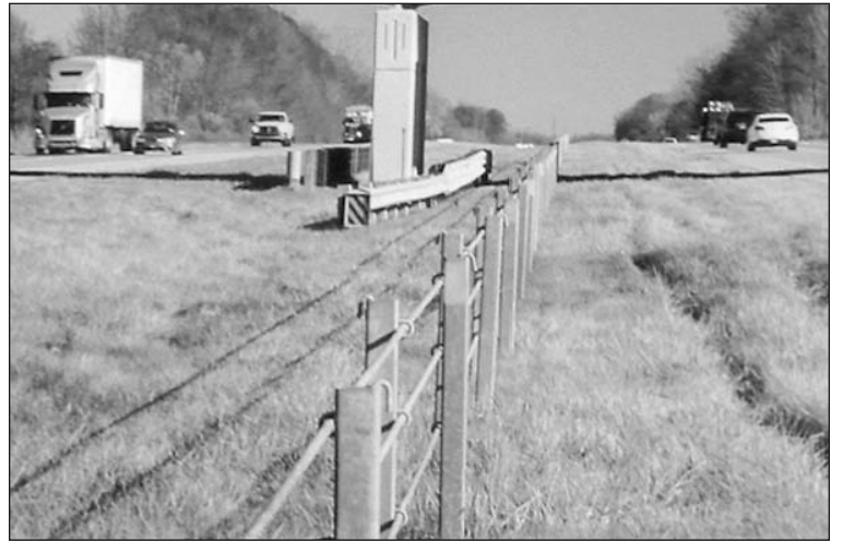
Cable barriers can stop crashing cars from crossing medians.
