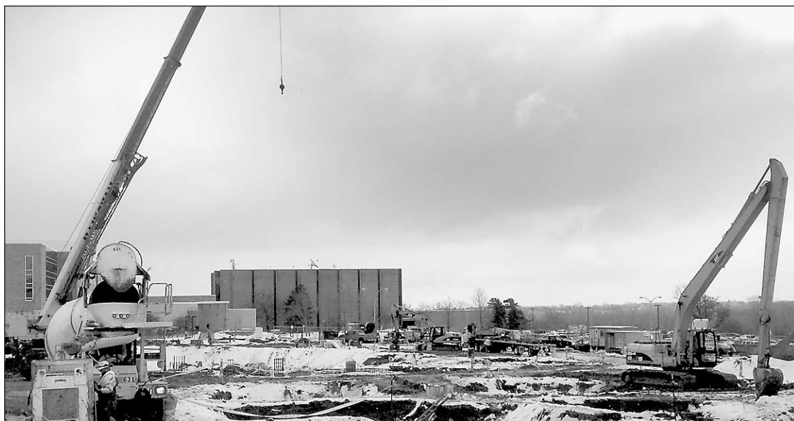
Construction of Oakland University's Engineering Center is underway.
