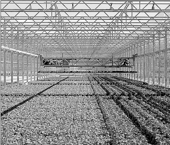
Instead of relying on natural gas, Metrolina Greenhouses uses waste wood from forest management and land clearing as an energy source in its 6.1M square-foot Huntersville, N.C., operation.
