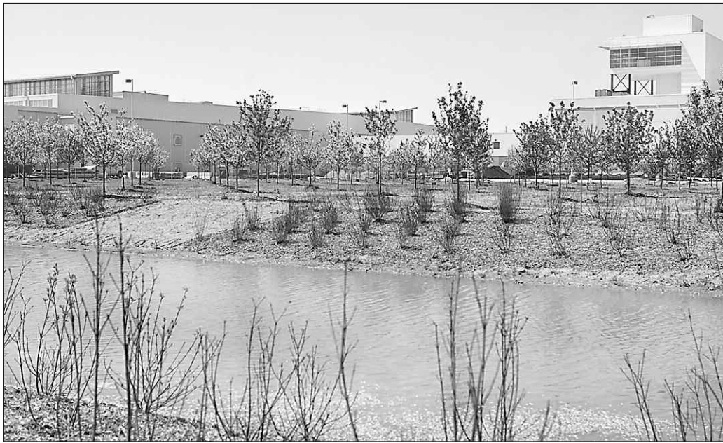
Retention ponds are the backbone of the Ford Rouge complex's elaborate storm water system. The Rouge site is now an image leader for Ford Motor Co.'s larger environmental "green" reputation.
